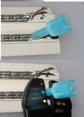
Slide on the appropriate male or female connector for this splice.
