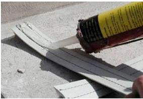
Apply E-Bond to the back of the E-Track paying special attention to the track ends where the connectors are. Apply a thin bead down the centre, skipping a few centimetres every 15 centimetres. For the best adhesion, press the track down to the surface so the E-Bond squeezes out towards the edges.
