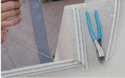
**E-Track** is delivered in 15 metre rolls. E-Track should be placed in position very near to where it will be secured to the surface using our **E-Bond**. E-Track will easily adapt to many surface imperfections and obstacles found on ledges and roof surfaces and is easily cut and joined to handle tight turns. Take the time now, before getting out the bottle of E-Bond, to make your cuts and corners.
